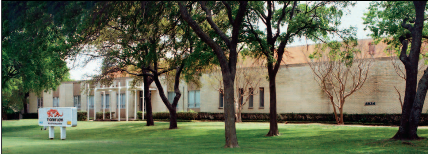
TIGERFLOW State-of-the-Art Headquarters, Manufacturing & NIST Test Facilities
